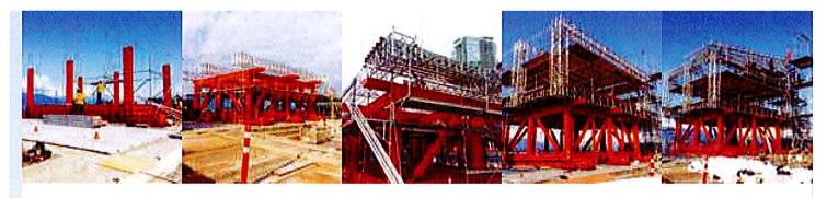
Engineering Services was able to design and engineer the temporary structure to meet all permanent structure requirements. Jenish Castello, lead scaffold designer for the project says "the structure was designed to 1/50 wind pressure, designed to seismic, 2.4 KPa & 1.2 KPa live load on deck levels (deck level 1 & deck level 2 respectively) and minimum roof live load of 1 KPa. "
