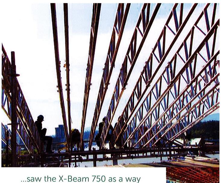
...saw the X-Beam 750 as a way to manage to hand build the structure while maintaining the high strength capability needed to reach seismic standards.
